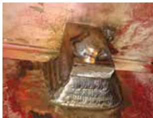
Pole stopper replaced during routine maintenance
