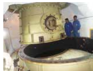
Partly removed Suction Cone Lower Part
