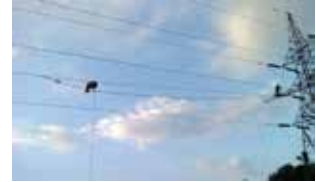
Live line maintenance of 220kV suspension tower
