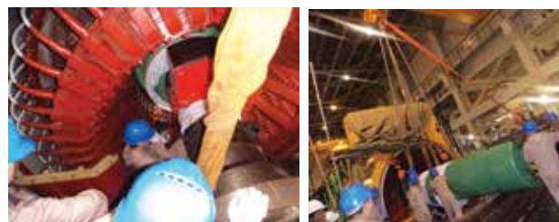
Extracting the Rotor of the Generator
