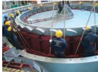
Lifting of the Generator Rotor
