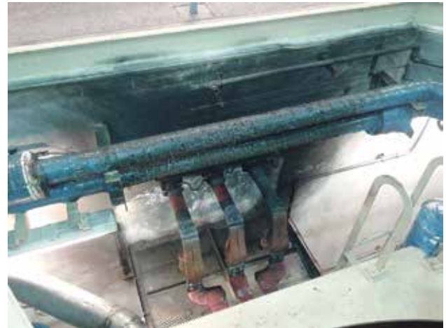
IPB Failure. (location- generator terminal)
