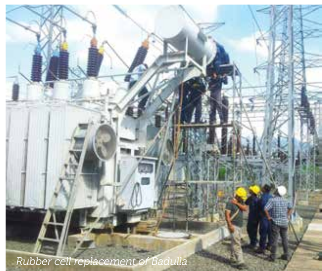
Repairing of pneumatic unit
