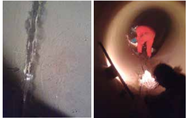
Penstock Defect Rectification Work at Old Laxapana PS
