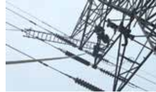
Live line maintenance of 132kV suspension tower
