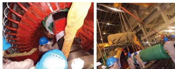
Extracting the Rotor of the Generator
