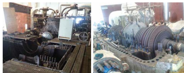
Lower Half of the Low Pressure Turbine
