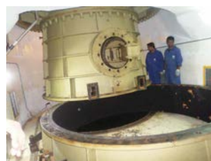
Partly removed Suction Cone Lower Part
