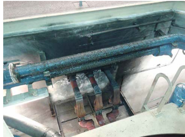
IPB Failure. (location- generator terminal)
