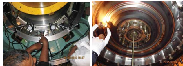
Inspection of Bearing Parts during Remedial Work of Samanala Wewa PS
