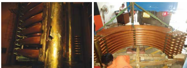
Breakdown maintenance of damages due to Thrust & UGB oil cooler leakage
