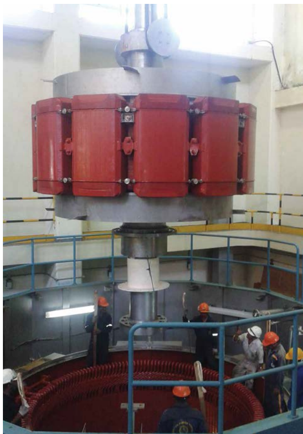
Generator Work during Major overhaul of Unit 2 of Canyon PS
