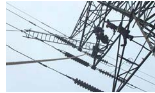
Live line maintenance of 132kV suspension tower
