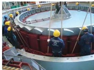
Lifting of the Generator Rotor
