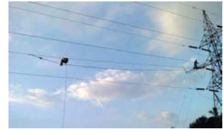
Live line maintenance of 220kV suspension tower
