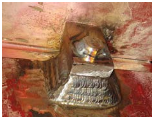
Pole stopper replaced during routine maintenance
