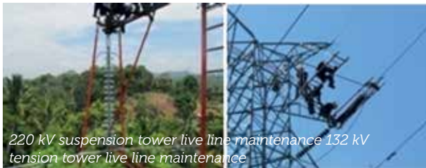
132 kV suspension tower live line maintenance 220 kV suspension tower live line maintenance
