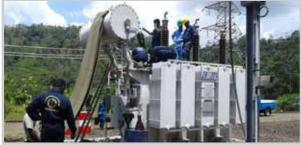
Servicing of tap changer of 10MVA Transformer at switchyard of KGPS
