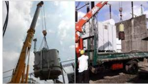
Replacement of defective single phase 250/3MVA 220-132/33kV Transformers at Biyagama GS
