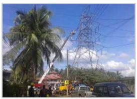
132kV Tower line - Insulator hot washing
