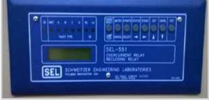
Installation of transformer protection relays (SEL 787 and SEL 551) was carried out by replacing existing electro mechanical relays.
