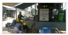
Oil Filtering of Kiibathkumbura Transformer
