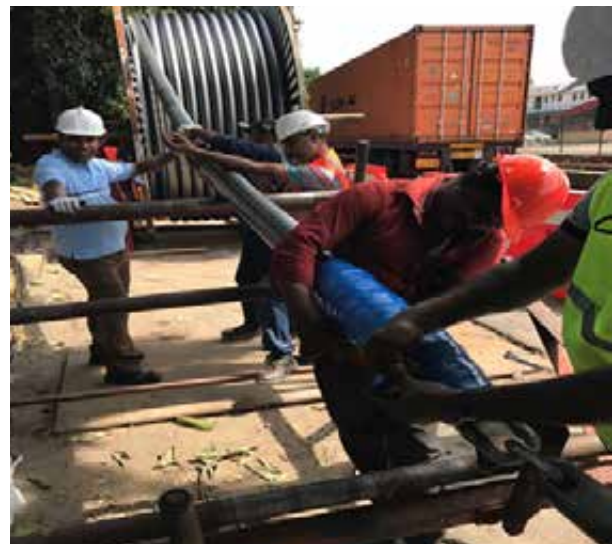
220kV Cable Pulling Work at Port Premises
