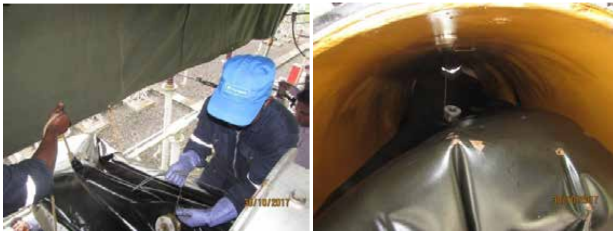
Canyon Unit #1 Transformer bladder replacement
