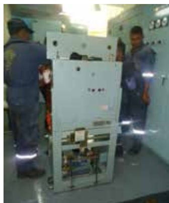
Canyon 12.5KV spare generator OCB overhaul works
