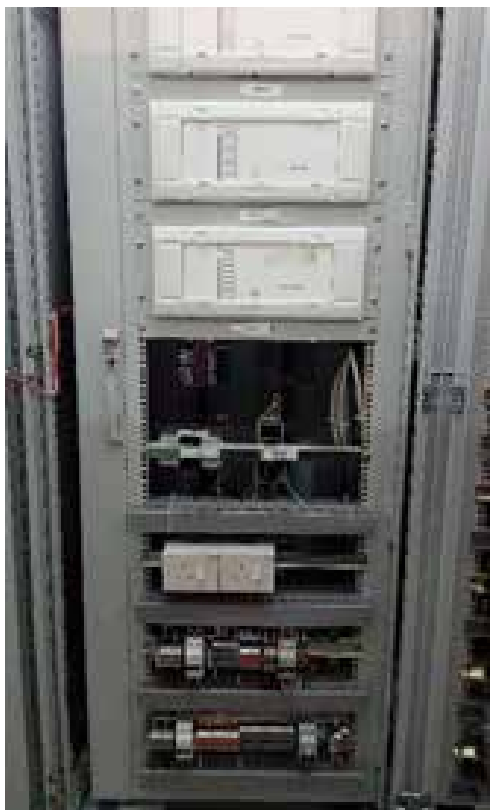
GE 264 RTU Installed at Rantambe Power Station
