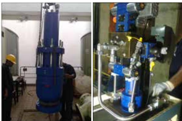
Retrofit of Turbine Governor of Kotmale Unit 01
