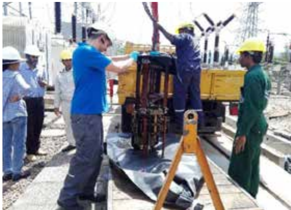
Disassembling a Diverter Switch at Rantembe switchyard
