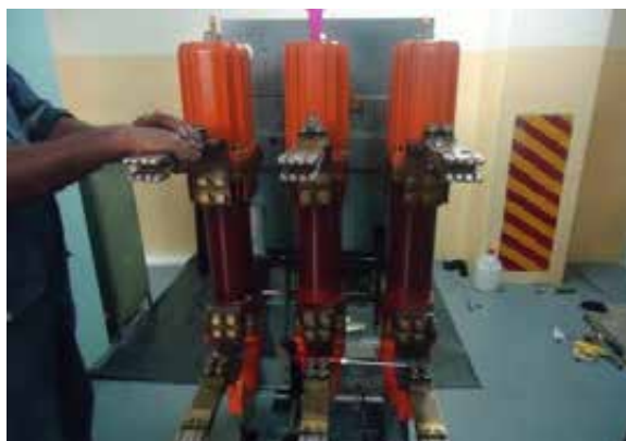
Canyon 12.5KV spare generator OCB overhaul works
