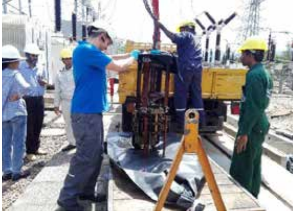
Disassembling a Diverter Switch at Rantembe switchyard
