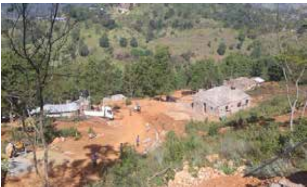
Construction of resettlement housing scheme of MHPP
