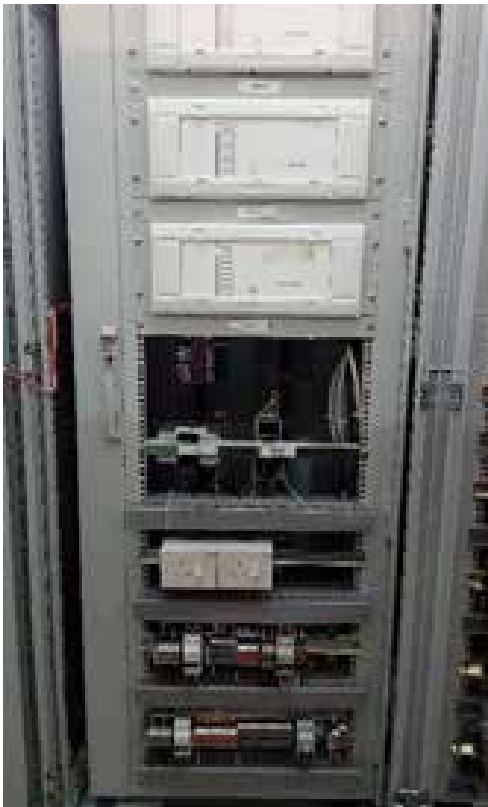
GE 264 RTU Installed at Rantambe Power Station
