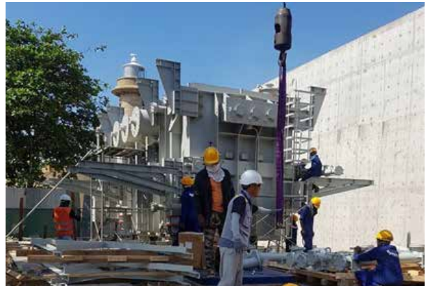
250MVA Transformer Installation Work at Grid Substation "L"
