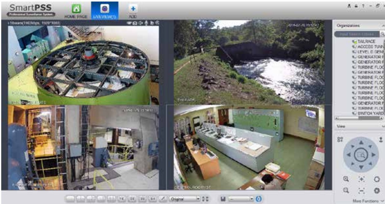
CCTV System Interface in Display Units
