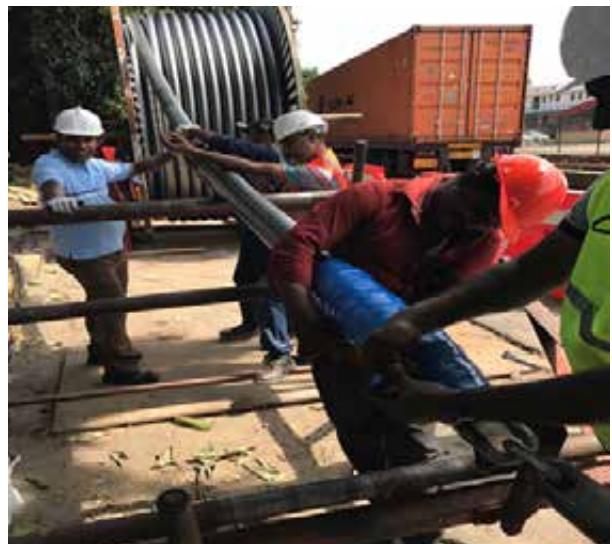
220kV Cable Pulling Work at Port Premises
