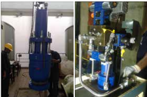
Retrofit of Turbine Governor of Kotmale Unit 01
