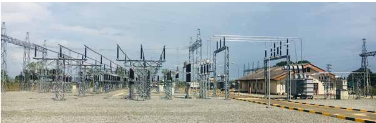
Hambantota Grid Substation Augmentation Work
