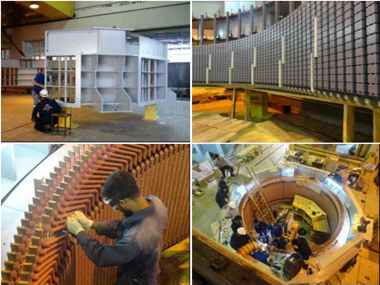
Refurbishment of unit # 1 is in progress
