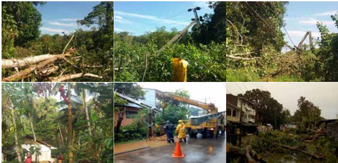
Power Restoration Due to Flood and Earth slip
