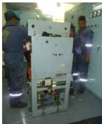
Canyon 12.5KV spare generator OCB overhaul works
