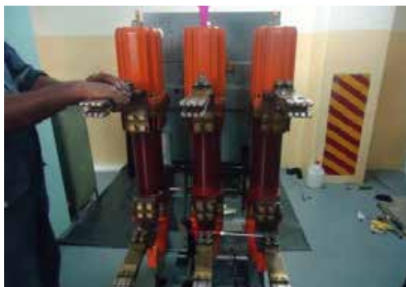
Canyon 12.5KV spare generator OCB overhaul works
