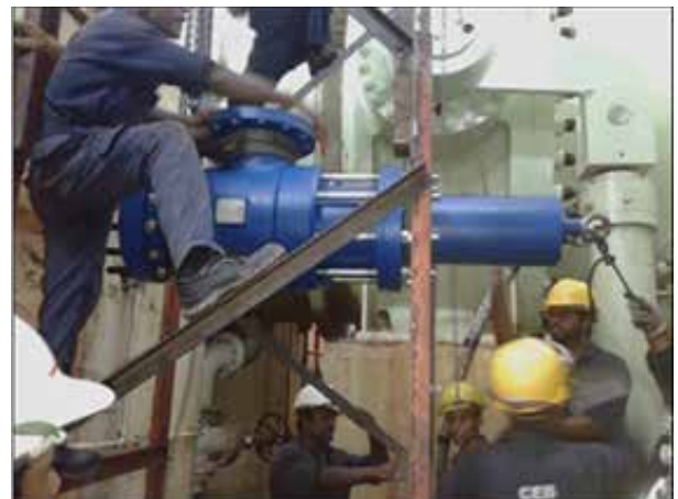
MIV Bypass Valve Replacement of Unit 01 Machine at Victoria Power Station
