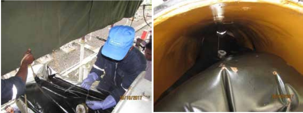
Canyon Unit #1 Transformer bladder replacement
