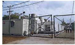
10 Nos.x1MW Diesel Generators installed at Kolonnawa Site
