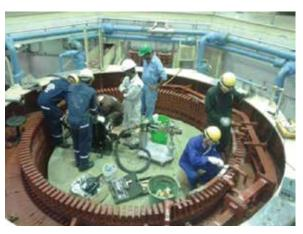
Soldering the replaced Stator Winding Bars in U-1 Generator
