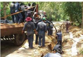
Replacement of Intake 11kV Power Supply Underground Cable at Victoria Power Station
