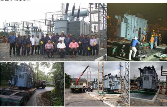
Figure 4: Installation of a new 31.5MVA Transformer at Pannipitiya GS which was shifted from Deniyaya GS.
