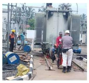
10MVA transformer at Old Anuradhapura GS was replaced with a 30MVA transformer transported from Old Galle GS after complete overhaul and assessment based on electro-chemical test results to improve the capacity of Old Anuradhapura GS.
