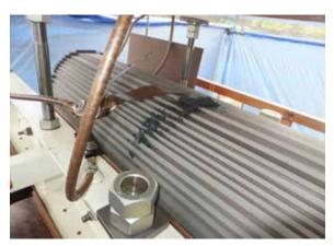
Repair the Core Earthing
