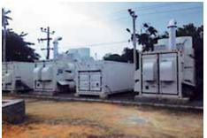
10nos. x1MW Diesel Generators installed at Thulhiriva
