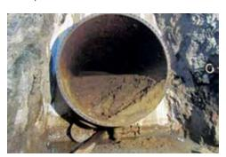
Silt deposited in the steel liner at Adit No. 1
