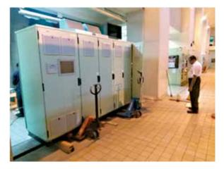
Replacement of AVR in Unit 01 and Unit 02 Machines at Victoria Power Station
