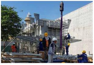
250MVA Transformer Installation Work at Grid Substation "L"
