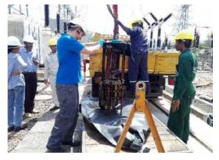
Dissembling a Diverter Switch at Rantembe switchyard
