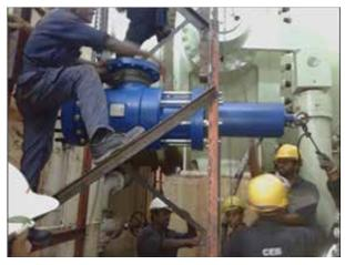
MIV Bypass Valve Replacement of Unit 01 Machine at Victoria Power Station
