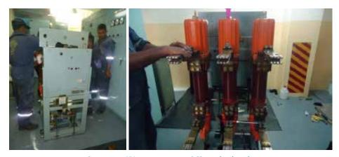
Canyon 12.5KV spare generator OCB overhaul works
