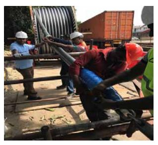
220kV Cable Pulling Work at Port Premises
