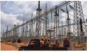
Figure P 7: 220/132/33kV New Habarana grid substation
