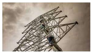
Figure P 5: Erection of 132kV transmission line
