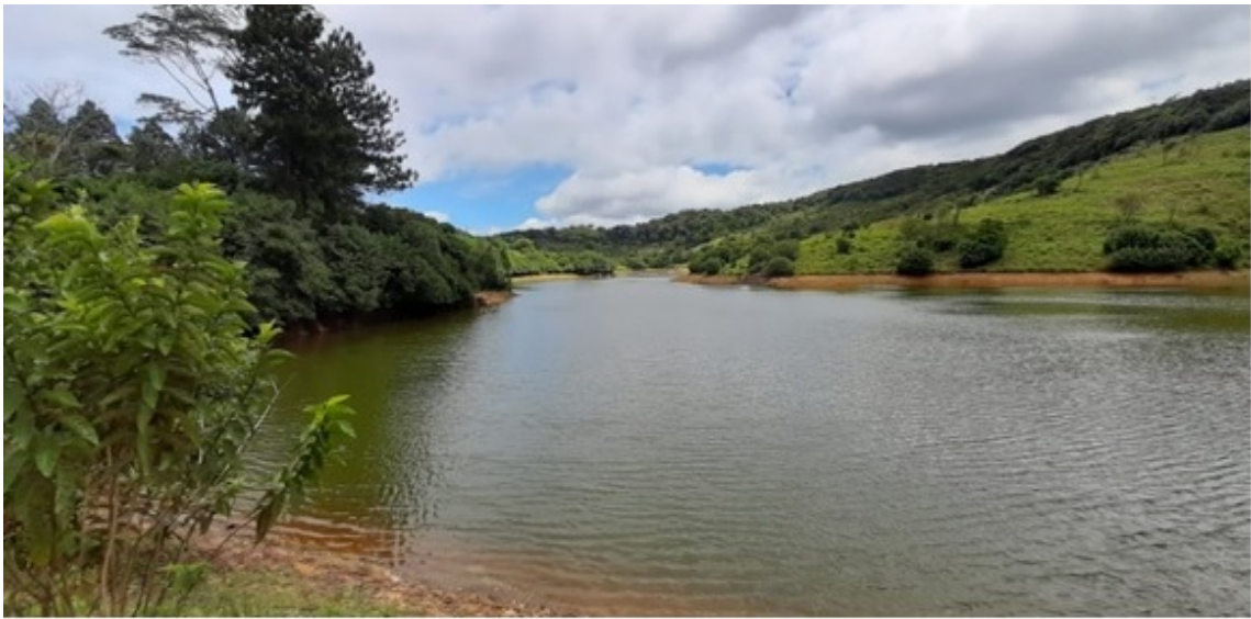
Figure 7-4: Photograph of Wewathenna Reservoir (Upper Pond)
